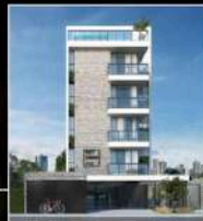
Key West 112 - Joinville (SC)
