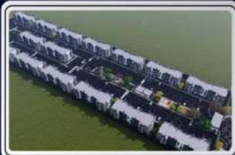
RESIDENCIAL HUBNER Joinville - SC Aprox. 19.140,66m 2
