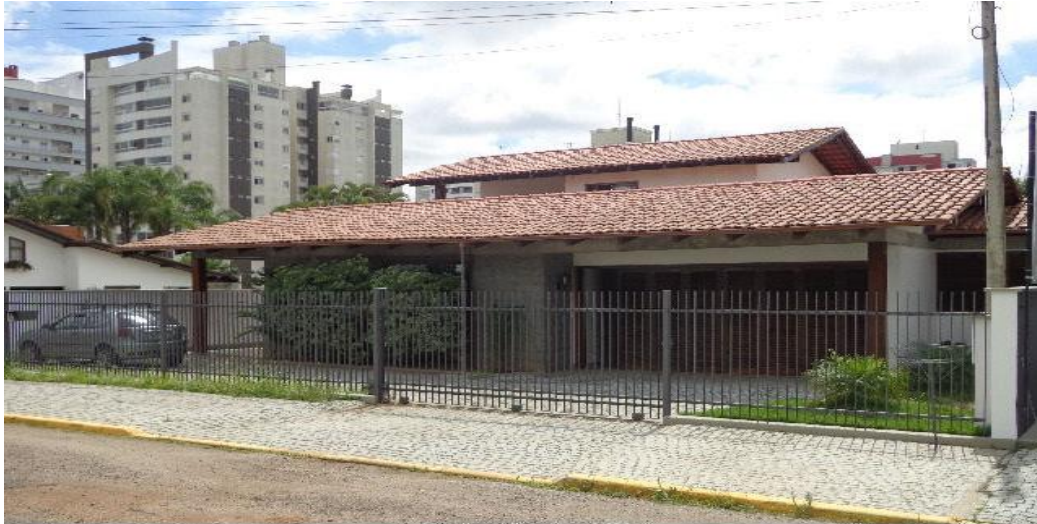
Rua: Camboriu, 200 Terreno 817,00m 2 Edif. 467,27m 2 Inscr. Imob: 13-20-12-93-36
