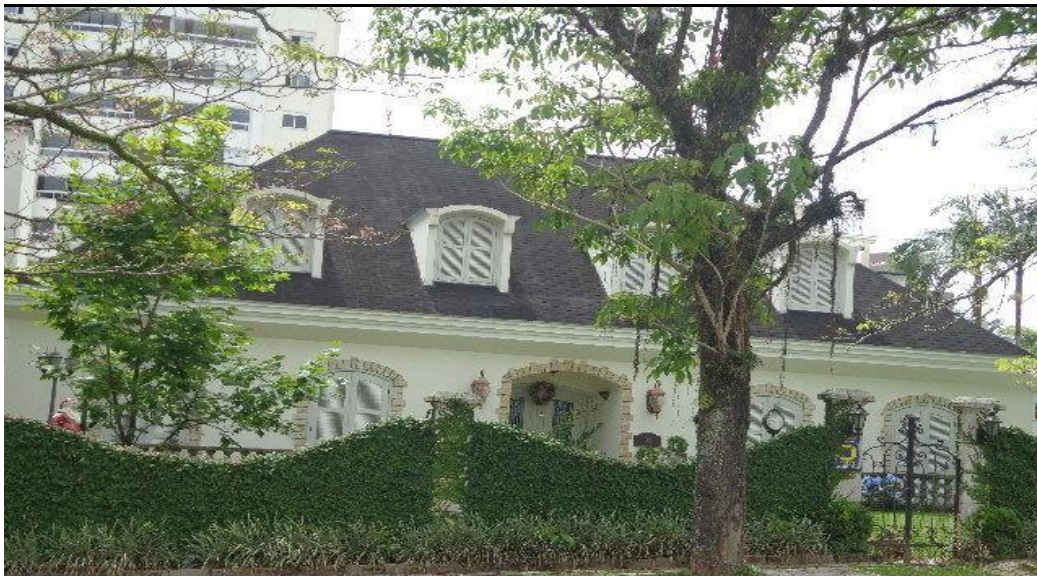
Rua: Camboriu, 98 Terreno 1.634,00m 2 Edif. 1,129,58m 2 Inscr. Imob: 13-20-12-93-131
